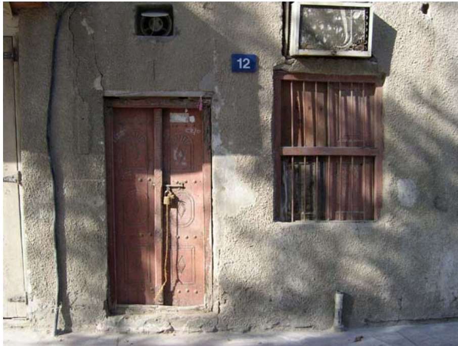
FIG. 19 old shop that is scheduled for renovation and re-use, Al Bastakaya, Dubai, 2004 (photograph by Ingram)
